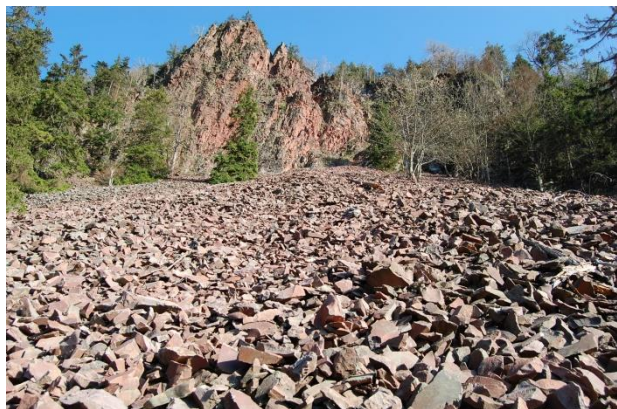
Figure 5 Contemporary activity of a scree slope at the foot of a landslide head scarp, Mt. Suchawa, Kamienne Mts.
