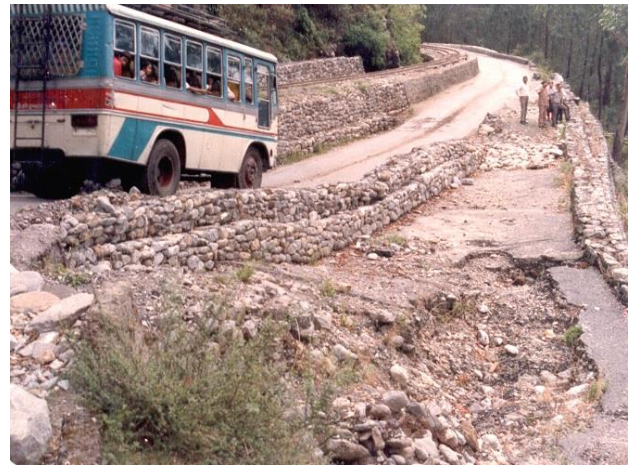
Figure 10 Recurring subsidence of the Hill-Cart road at Pagla Jhora, where the tourist traffic to Darjiling has been badly affected (Photo: Author)
