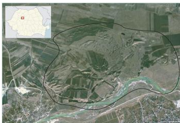
Fig. 1: Localization of the studied deep-seated landslide
