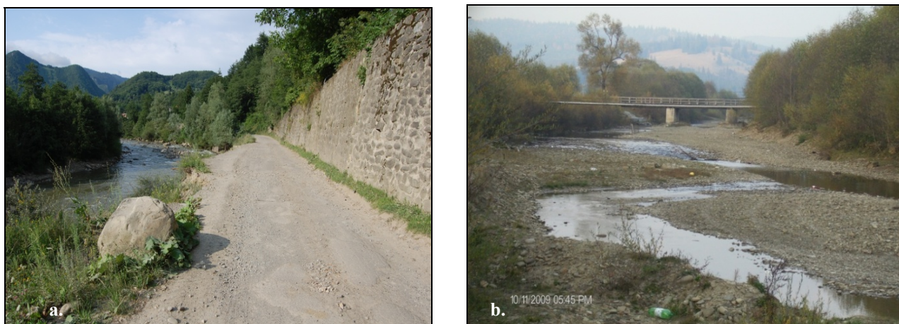
Fig. 6. Geomorphological effects of floods on the Bâsca River channel: river bank erosion (a) and alluvial processes (b) (Photo: Minea, November 2009).
