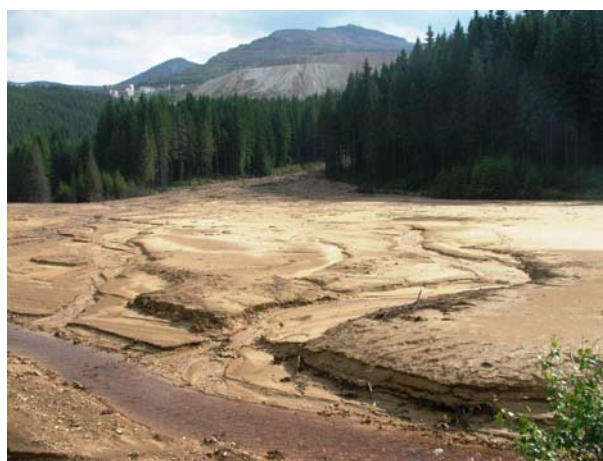
Figure 5. Hyperconcentrated and debris flow deposits accumulated behind the Pinul dam
