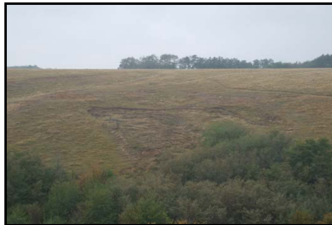
Photo 2. Landslides on the left slope of the Valceaua valley, Sacel, Santamarie Orlea commune (October, 2010)
