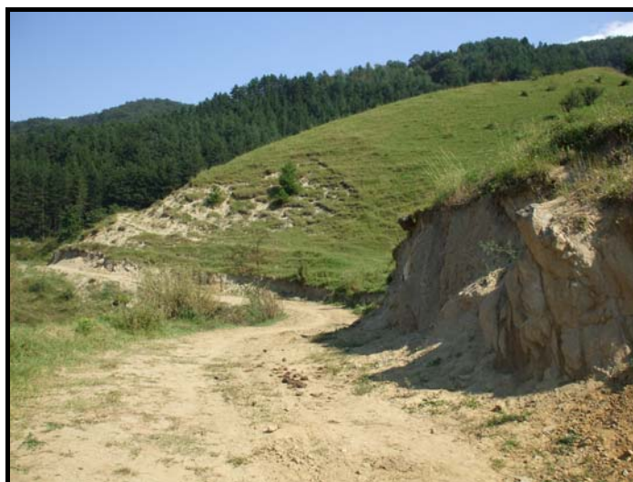
Photo 4. Landslides and erosion processes on the right slope of the Strei valley, Ponor, Pui commune (August, 2010)
