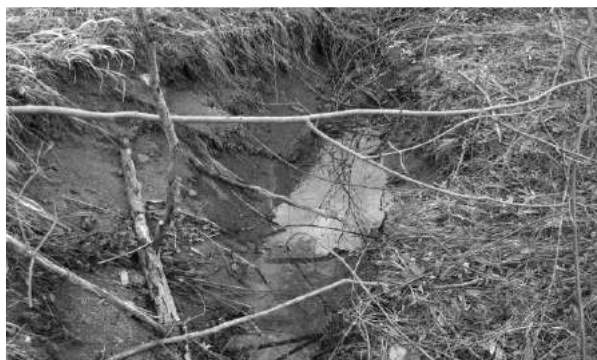
Fig. 9. Pond formed in a transverse crack
