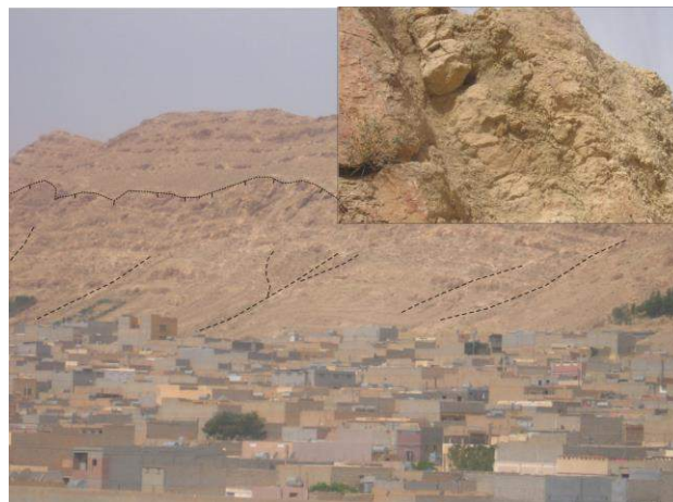
Fig. 2b. Slope-related hazards
