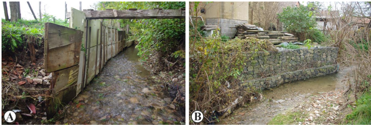
Photo 6 Simple makeshift bank revetment (A) and gabion protection (B) of banks (Photo by P. Kalmár 2014)
