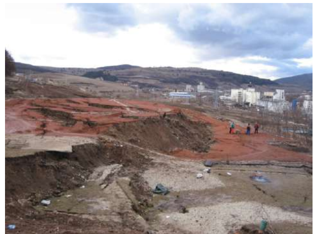
Figure 11 Landslide in a recreational park, 2016
